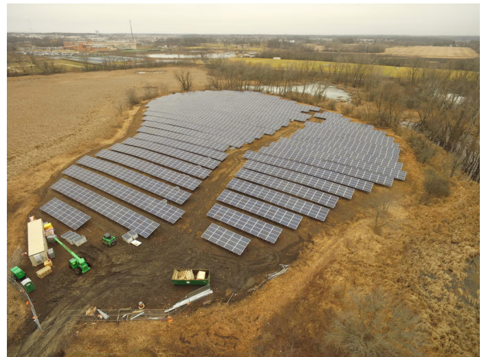
Grayslake High School District 127, solar panels financed by Wintrust Government, Non-Profit & Healthcare group.
